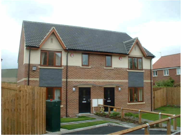
New high quality home in Morrith Close in partnership with Yorkshire Housing (official opening 10 th May 2010)
